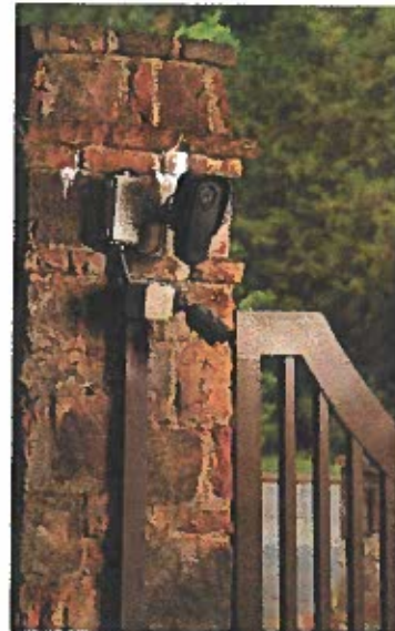
Electric & Existing Structure / Pole
